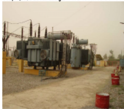
Photograph 1 Subproject 2 Bahawalnagar ITC 40MVA transformer.
