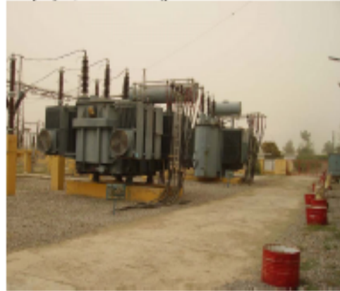
Photograph 1 Subproject 2 Bahawalnagar ITC 40MVA transformer.
