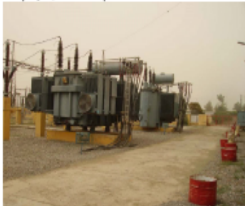
Photograph 1 Subproject 2 Bahawalnagar ITC 40MVA transformer.
