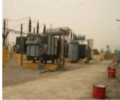
Photograph 1 Subproject 2 Bahawalnagar ITC 40MVA transformer.
