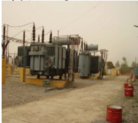
Photograph 1 Subproject 2 Bahawalnagar ITC 40MVA transformer.
