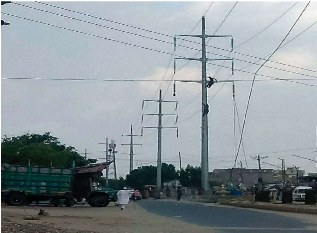
Newly Constructed 132KV Transmission Line for Zehnfa Powerhouse Chobara
