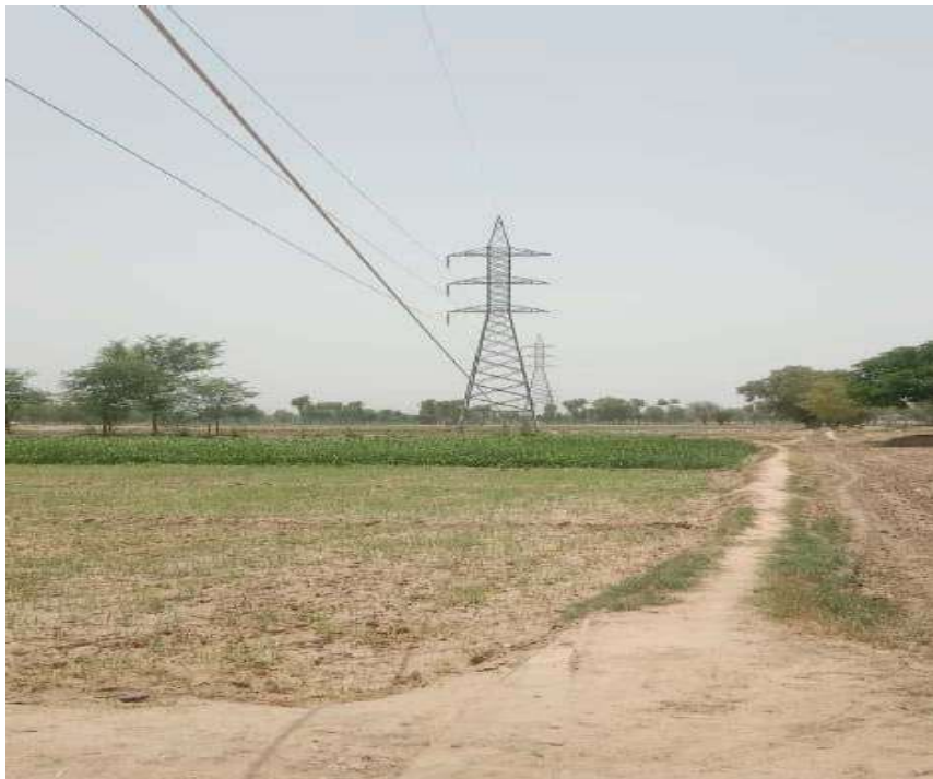
Newly Constructed 132KV Transmission Line 500KV RYK Sardar Garh to 132KV Feroza.
