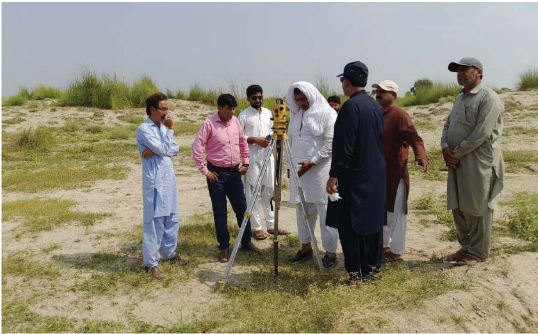
Demarcation and Possession of state land procured for 132KV New Grid Station Shah Jamal
