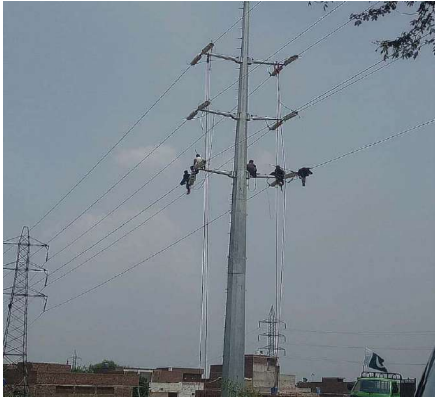
Work at 132KV Transmission Line in progress.
