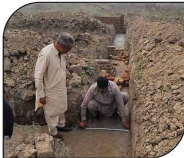
Civil Works in progress for New 132 KV Grid Station Pak Pattan II.
